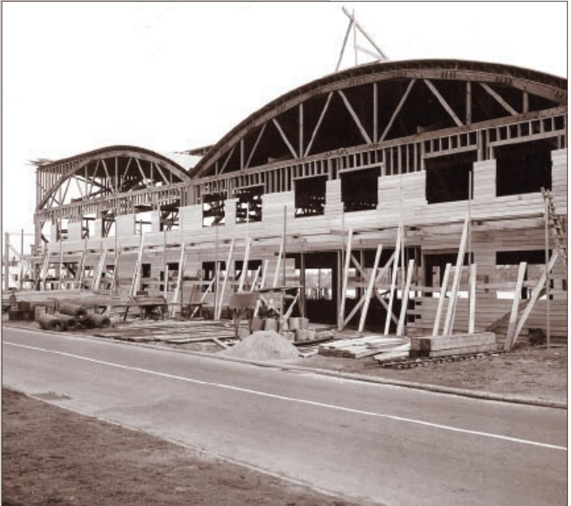
*Esther Sonnenberg noted: “When the plant was still on the drawing boards, Chet battled with the architects/engineers and finally won out to build it a foot higher off the ground — at considerable cost. Several years later that extra foot kept our plant from flooding, while those down the road did.” This building stands today as part of a much larger plant, which has grown from 10 to 75 acres and 750,000 square feet under roof.*
